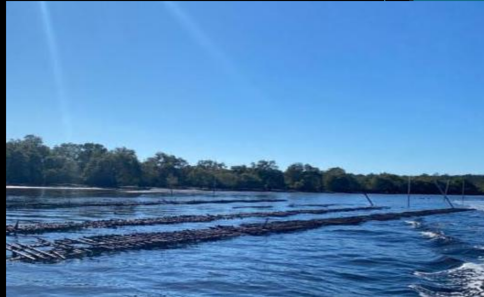
Neat and Tidiness/Structural issues
