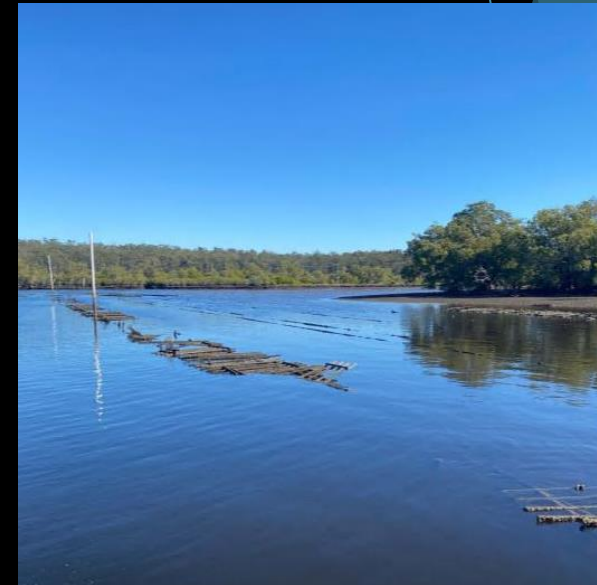
Intermediate markers/structural damage
